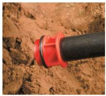
**5. Insert Fully Installed**Tap insert fully (up to the shoulder of the insert) into the pipe using a flat object.
