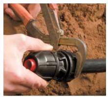
**8. Tighten Nut with a Wrench**The nut must then be tightened with a wrench.
